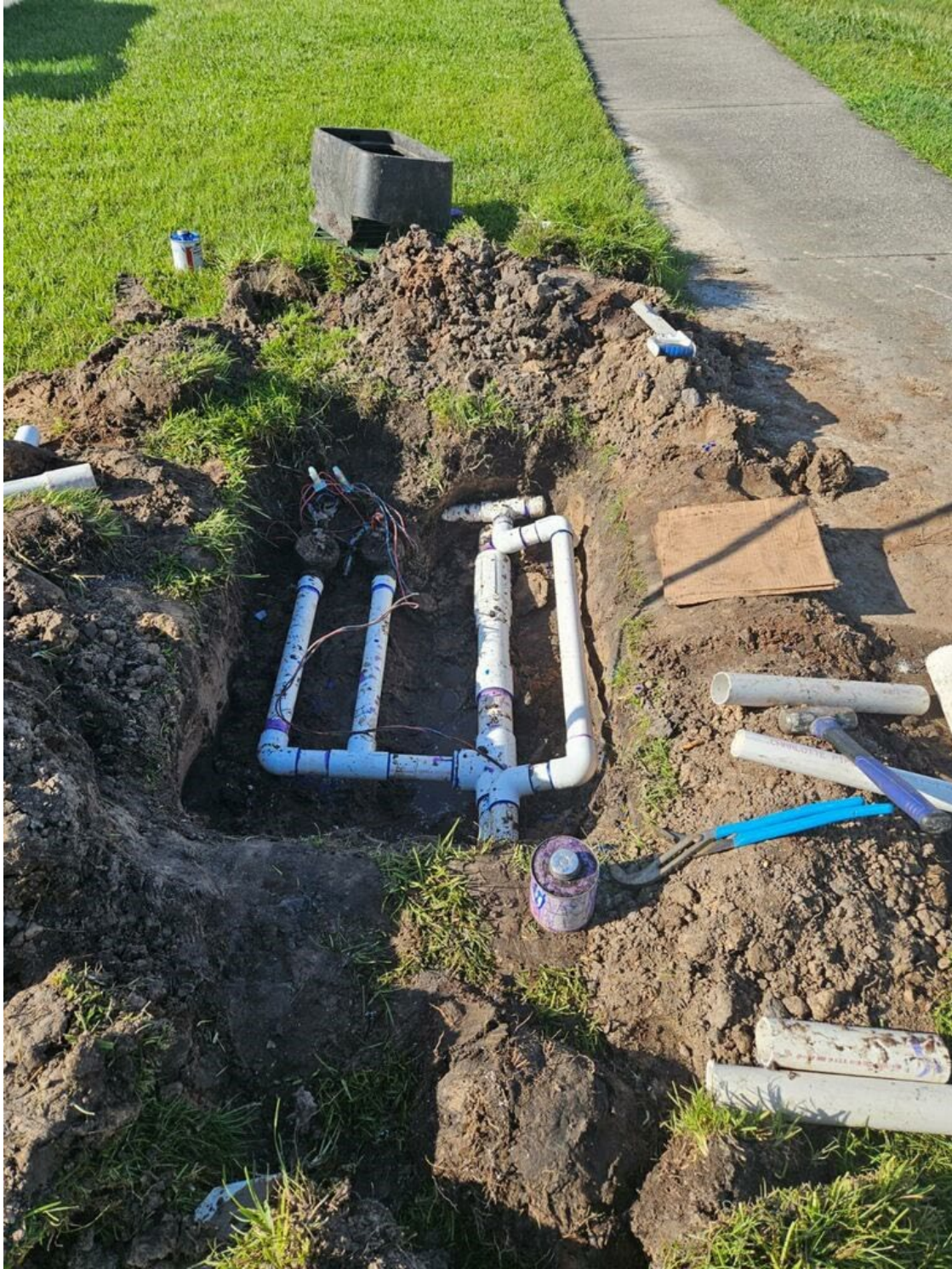
Completed mainline repair at valves 36 and 37.
